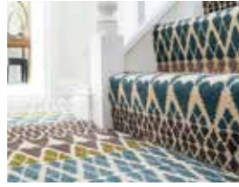
Private Villa, Abu Dhabi Installing carpet flooring
