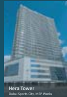
Hera Tower Dubai Sports City, MEP Works
