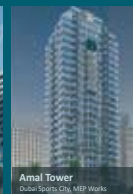
Amal Tower Dubai Sports City, MEP Works
